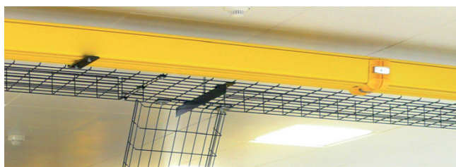
Typical installation of an overhead tray with ceiling mounted supports
