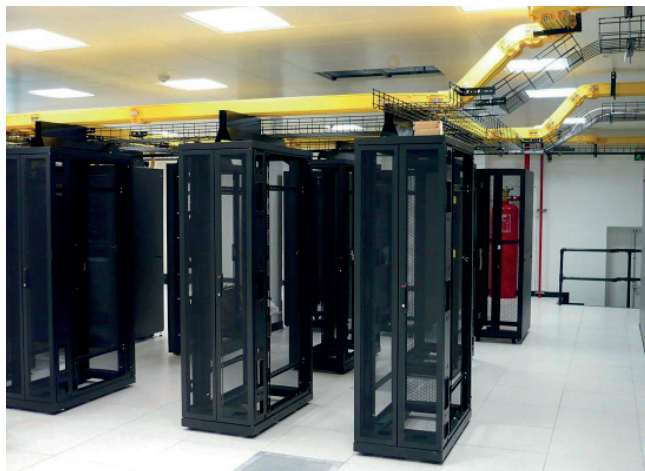
Typical installation of overhead copper and fibre management system with customised brackets to the top of the cabinets
