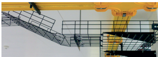
Typical installation of an overhead tray with brackets and support angles
