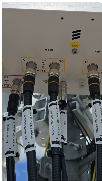
Jumpers identification under antenna
